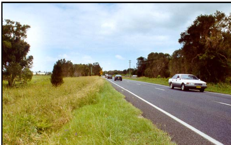
PHOTO 1: View of Ewingsdale Road looking east towards Byron Arts & Industry Estate [left background]. Site access would need to be provided off this busy road.
