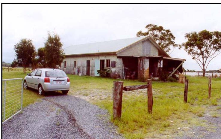
PHOTO 4: View of existing cottage [under current lease] looking north-west. Works are in progress on adjoining West Byron Effluent Reuse Wetland site [background].
